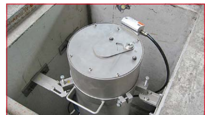
IR camera in a special protective housing for measuring after pressing
