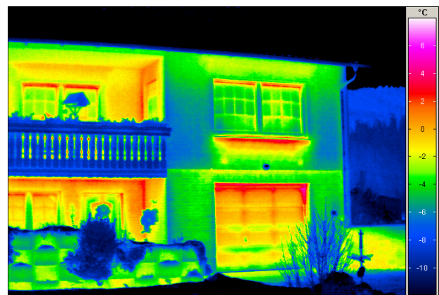
Heat loss below the window and at the door of the garage
